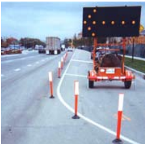
Properly placed channelizing devices and arrowboards are important in providing drivers with a clearly defined travel path.
