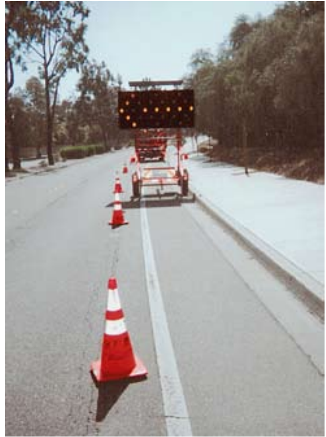
Lane closures help shift traffic away from the construction area to better protect the workers, and the drivers.
