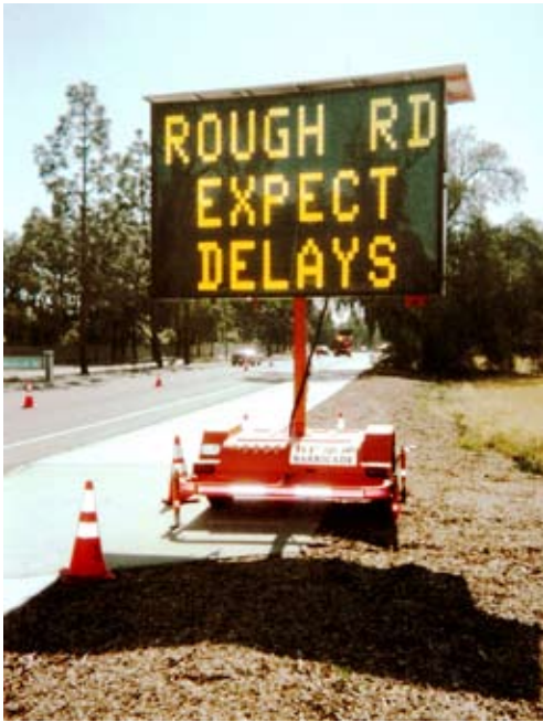
Message boards help explain traffic changes & delays to the motoring public.
